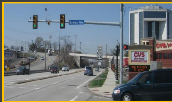
Adaptive Signal Control Technology
