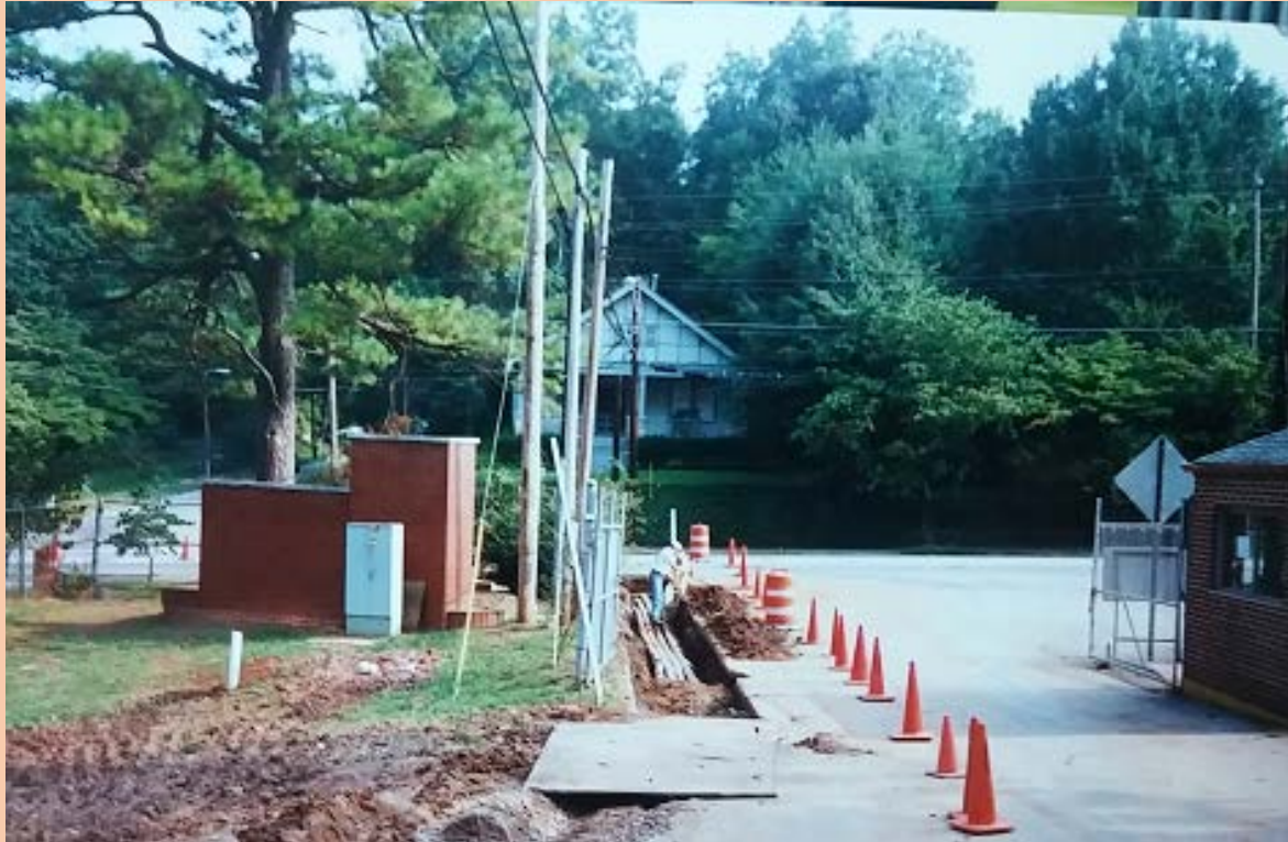
Pic showing trunk fiber coming in from street
